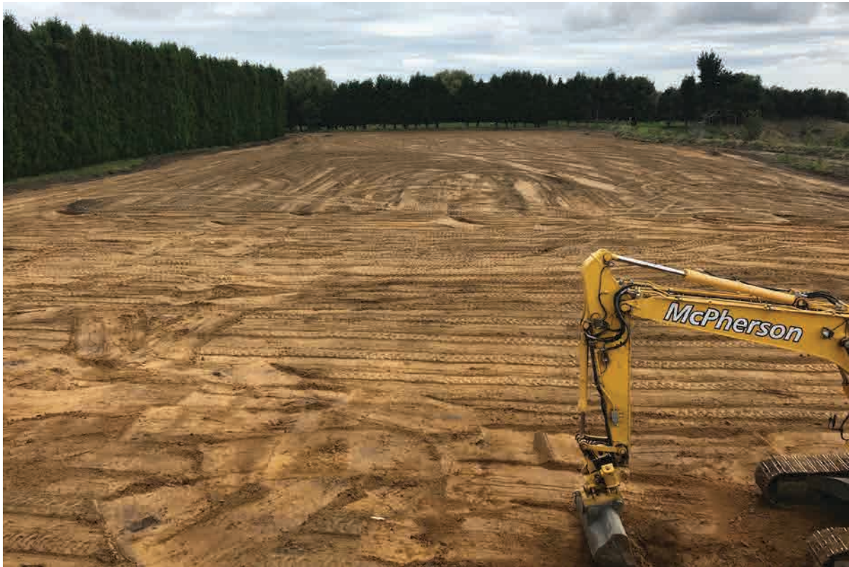
Figure 10. View south of 81B Kennedy Road post topsoil stripping.
